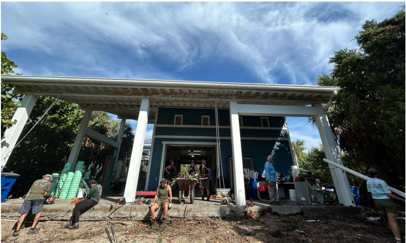
Tampa Bay Watch staff work together to repair building damage after Hurricane Milton. Photo credit: Tampa Bay Watch
